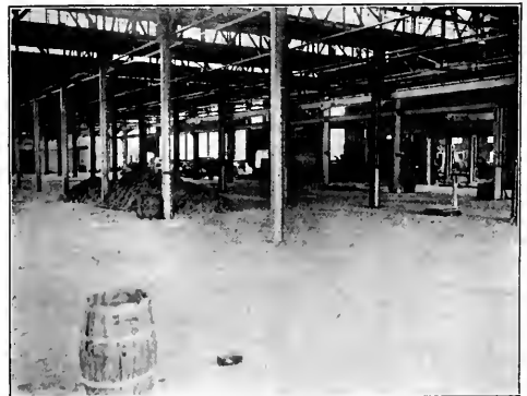
Cut 1—Lunkenheimer New Ferrous Foundry Building, Ready for Occupancy March 24, 1917.
